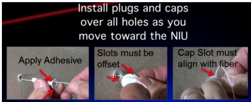
4.5.11 Install wall plugs and caps as you reach them, working the slack toward the ONT.
